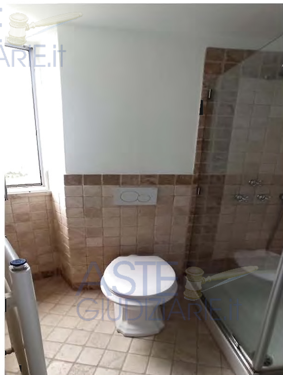
Vista locale wc 3
