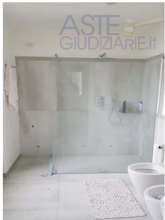
Vista locale wc 2
